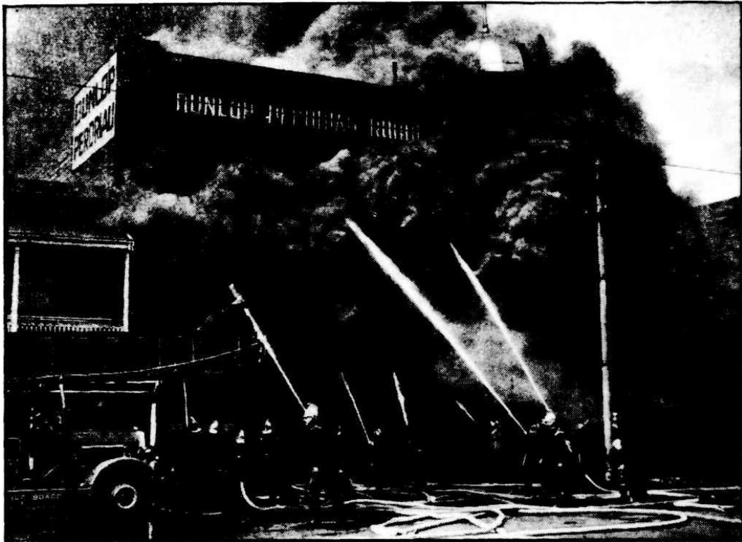
THE FIRE which destroyed the warehouse of Dunlop Perdriau Rubber Coy., in Flinders street, Adelaide, yesterday, was the worst for 17 years, total damage being estimated at £120,000. All brigades in the metropolitan area were summoned. This was one of the most spectacular blazes seen in the city.
